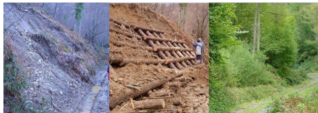
Landslide stabilisation in Forestry -P. Sangalli
